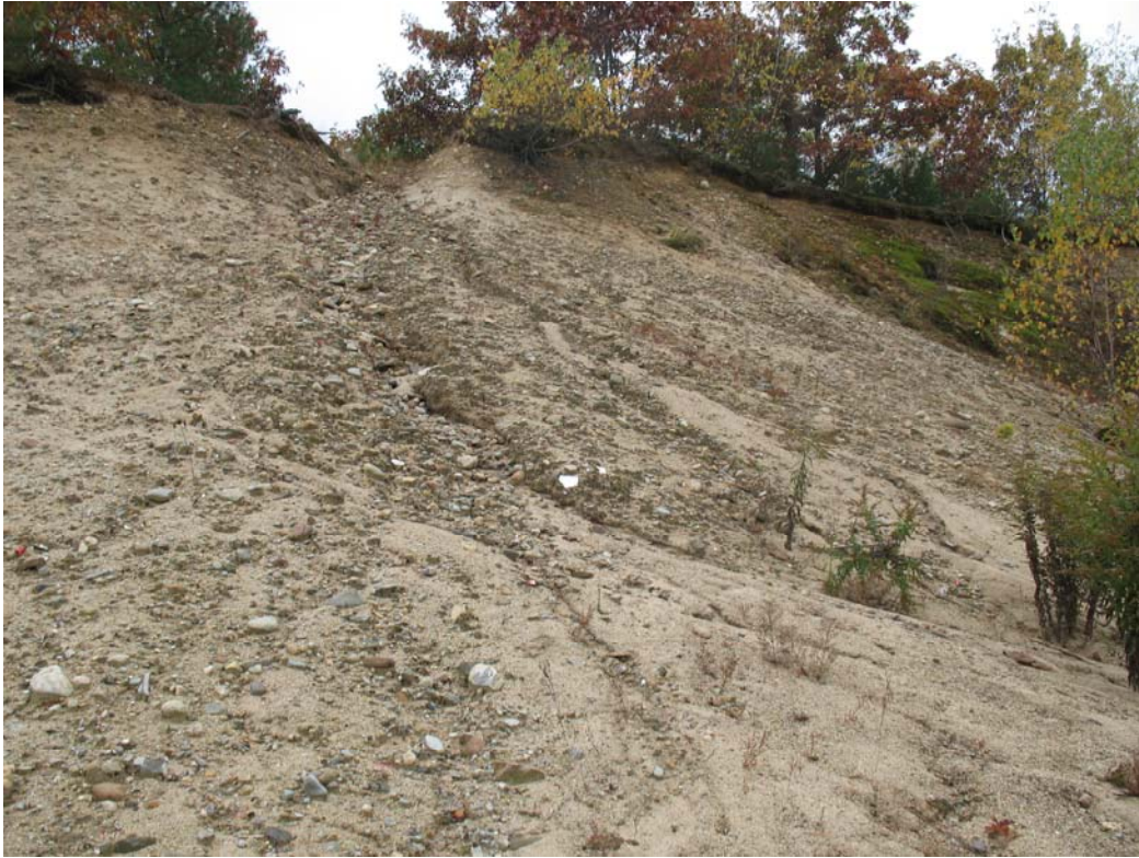
Photograph No. 7 (taken 10/16/13): View of erosion continuing on existing sand esker slopes southwest of the muck moat.
